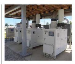
on input command of DO, pressure, or flow control. The MCP gives the plant SCADA system one point of contact for all blower data, aeration control set points, and control process data. Likewise, it manages starts, stops, and speeds for all of the blowers.
