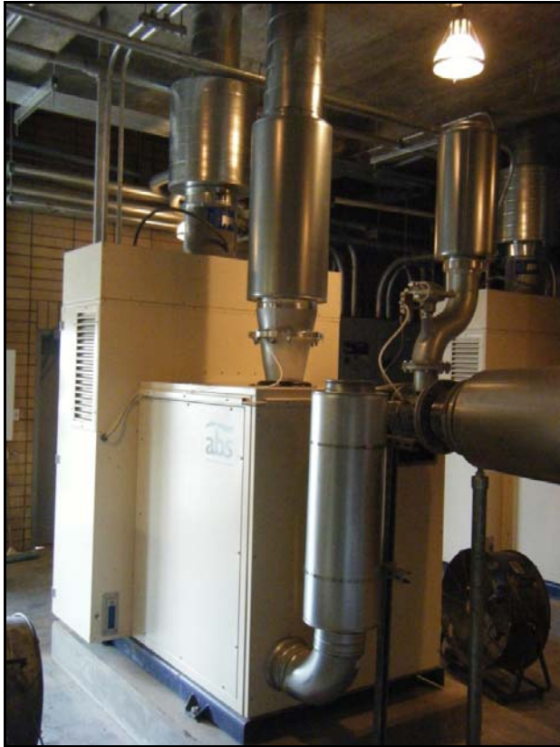
Figure 6. High speed turbine blowers installed for a new activated sludge system. The new blowers were combined with the existing blower control system after several integration challenges were overcome.
