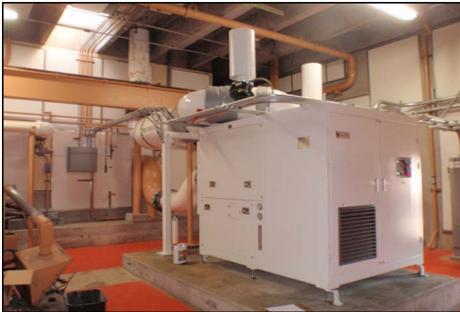
Figure 1. Twin core and dual outlet manifold turbine blower installation. Note the dual silencers projecting up from the discharge manifold.
