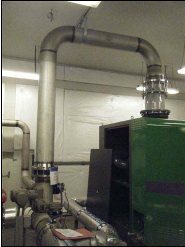
Figure 5. Blower outlet piping without a standard blow-off valve to provide a low pressure start-up condition.
